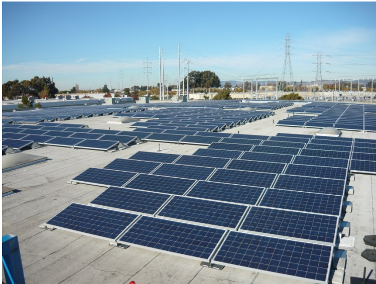
PV Rooftop Installation
